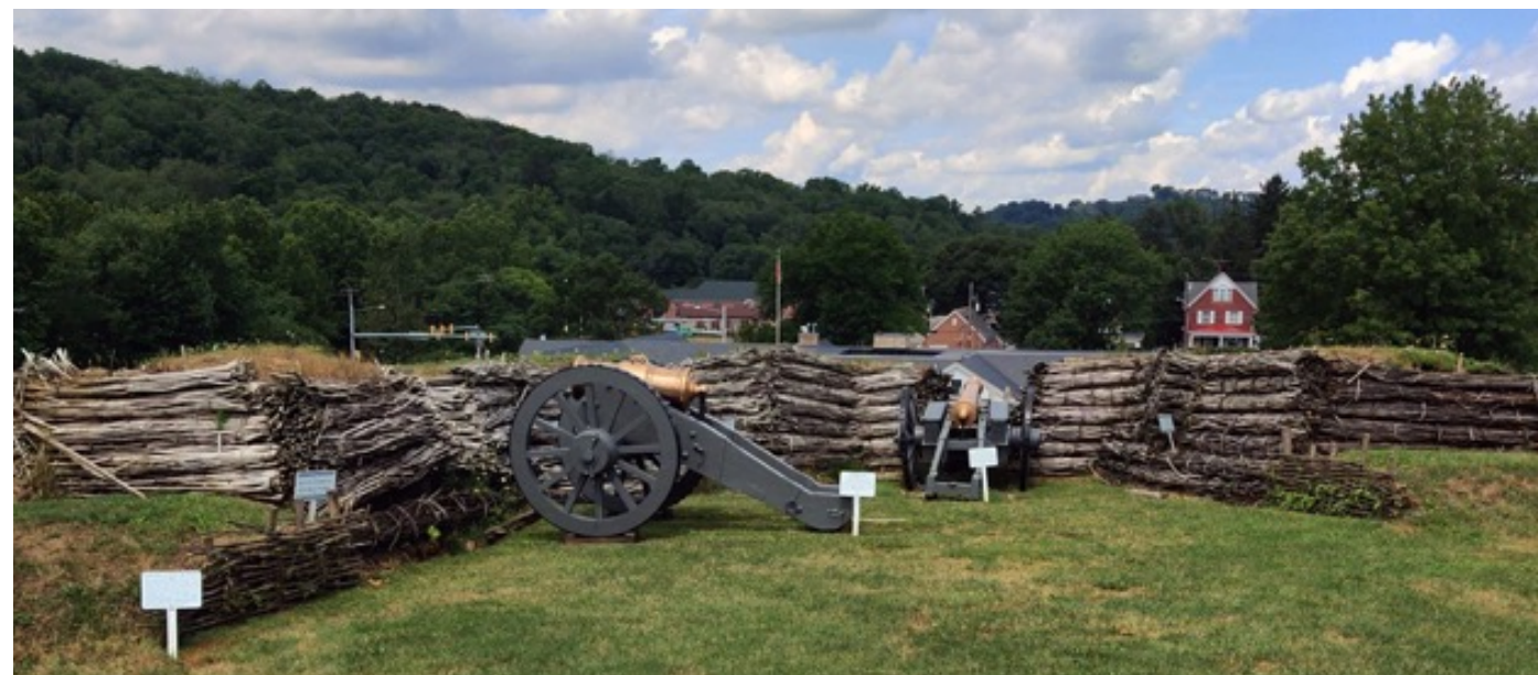
An example of fascine at Fort Ligonier. A cylindrical bundle of small sticks of wood, bound together, used in raising batteries, filling ditches, strengthening ramparts, and constructing parapets.
