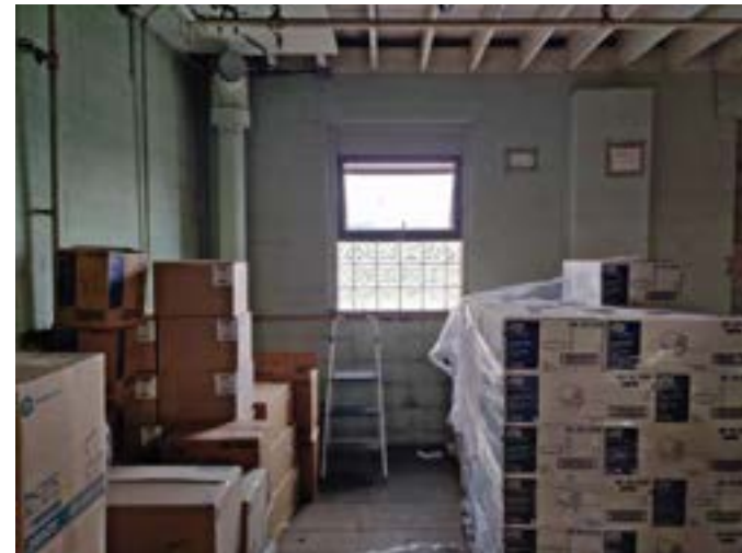
Cinder block construction of the warehouse.
