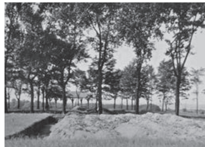
Trench excavations 30" in depth located part of the Pest House foundation and evidence of the 1795 east blockhouse.
