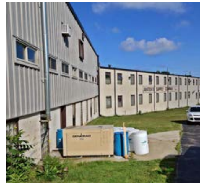
East view of Janitor Supply warehouse.
