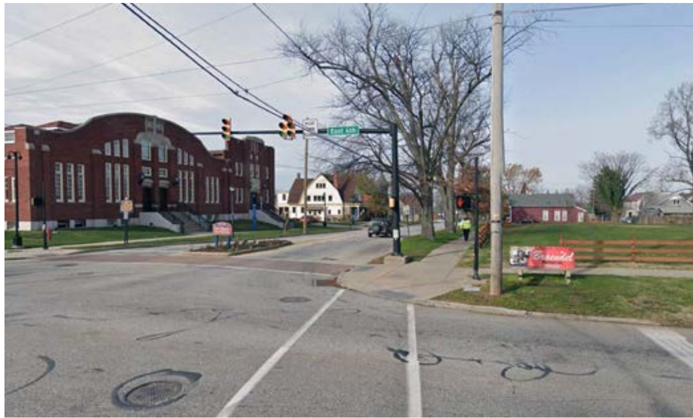
Main access into the Historic East Bayfront neighborhood is the intersection of E. 6 th Street and Parade Street. The Erie Armory is a prominent restoration effort made possibly by Erie Insurance that welcomes residents and visitors to the community.
