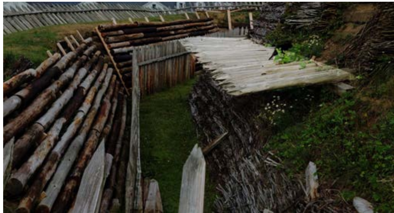
Fraises lodged in the parapet above the ditch and escarpment at Fort Ligonier
