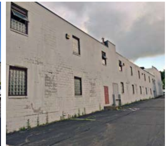
West view of Janitor Supply Warehouse
