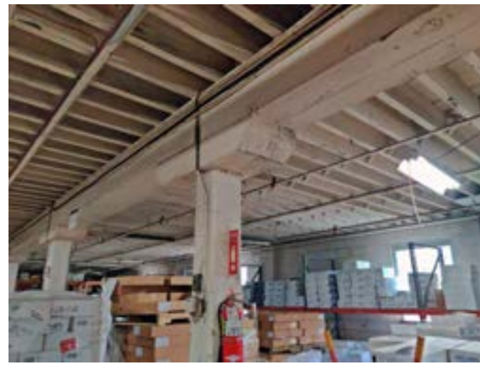
Interior view of post and beam construction.
