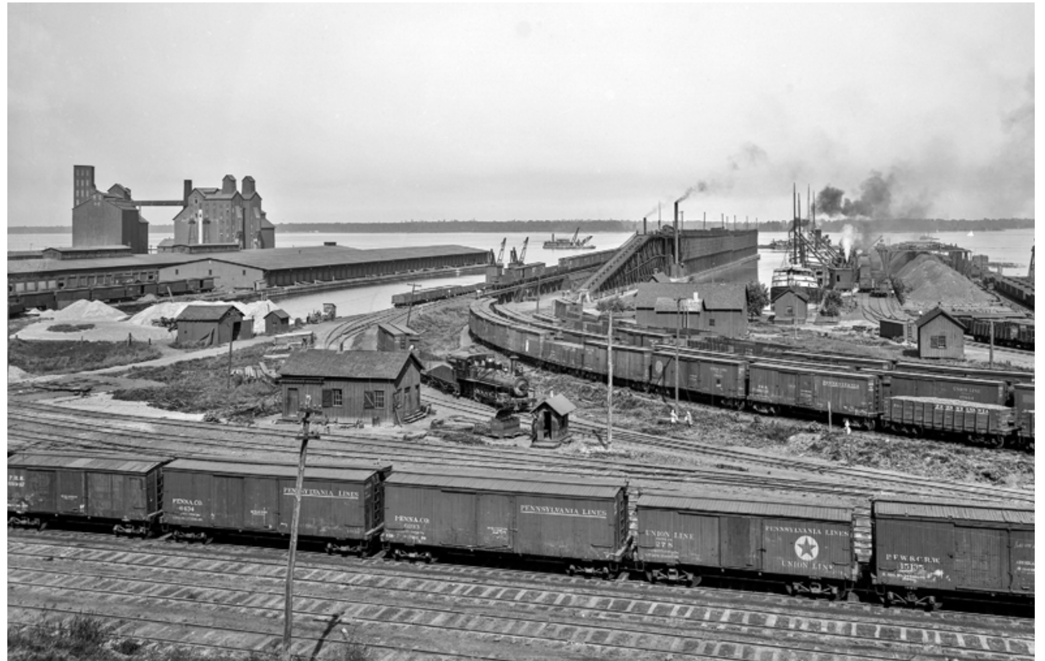
Anchor docks below Front Street, c. 1910
